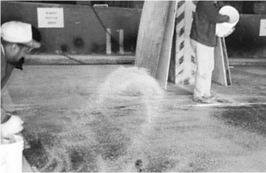
Aggregate is “broadcast” into wet resin
